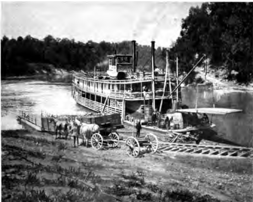
BURNSIDE LANDING, BURNSIDE, KENTUCKY.
